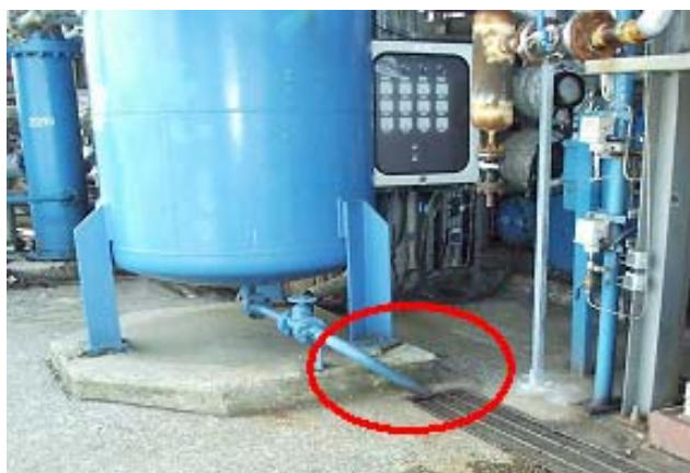
Figure 5 The site of the incident; with the vent red ringed
