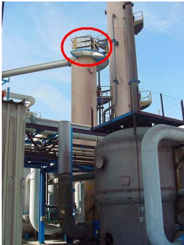
Figure 4: The tower after completion of the work
