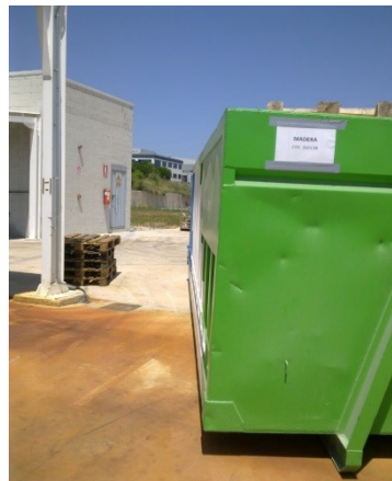
Figure 6 Properly labelled and segregated waste container
