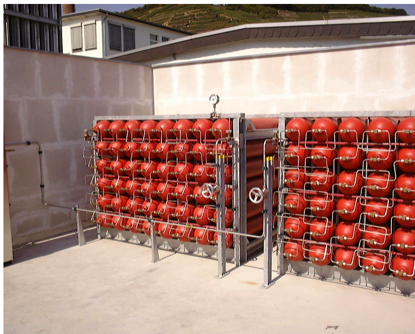
Figure 12: Typical High-pressure bundles.
