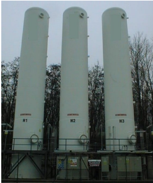
Figure 13: Medium Pressure Storage vessels (gaseous hydrogen)
