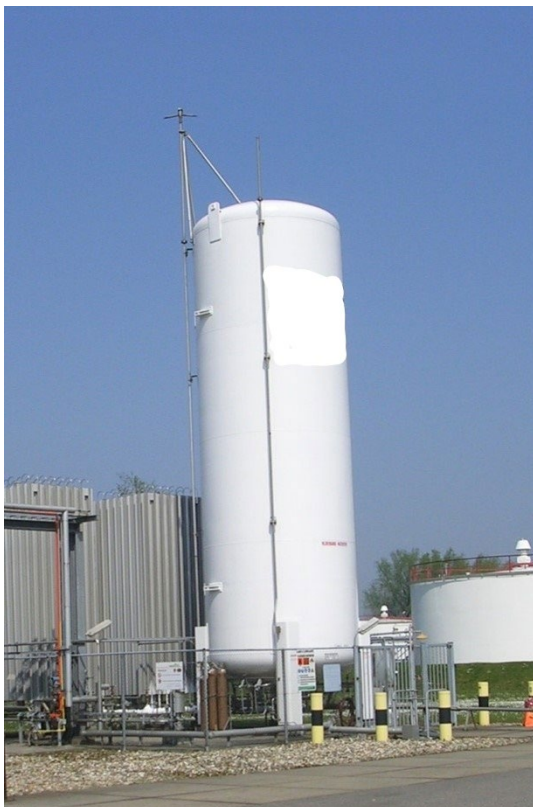
Figure 15: Typical LH 2 Cryogenic tank
