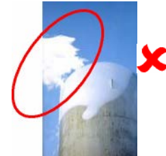
This picture shows gas venting from a vacuum protection device
