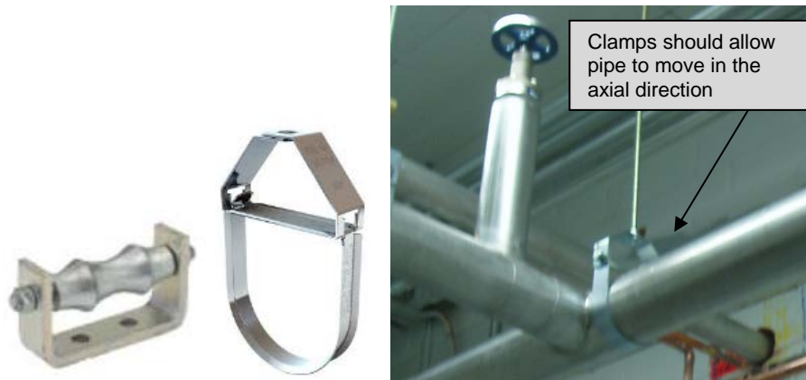
Figure 10 Examples of hangar and roller supports
